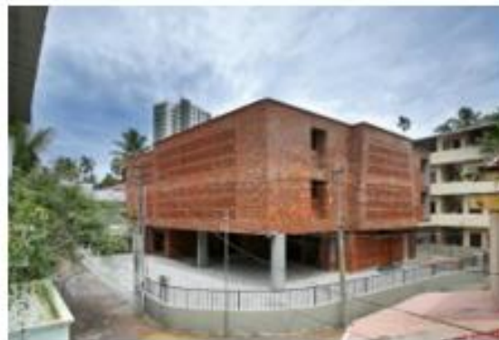
Figure 1: The double-slanted louvered brickwork facade of the Benziger Hospice Home by Srijit Srinivas Architects, showing a glare-free, non-institutional identity.
